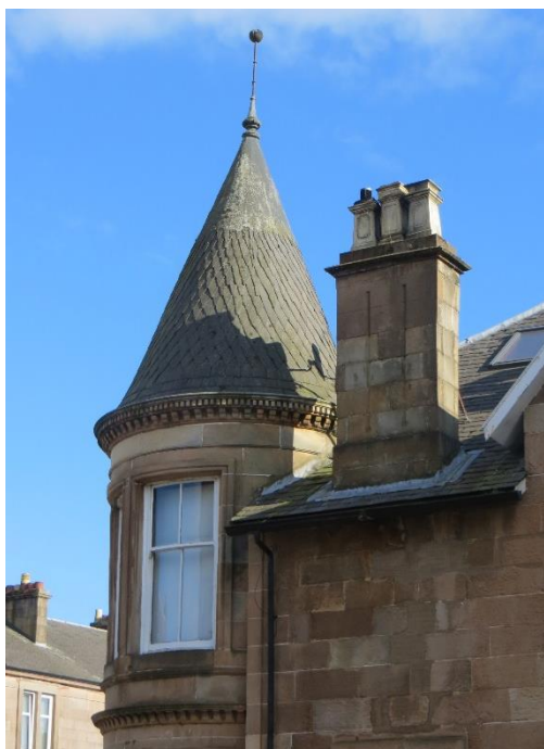
Figure 13 Turret with fishscale patterning and finial
